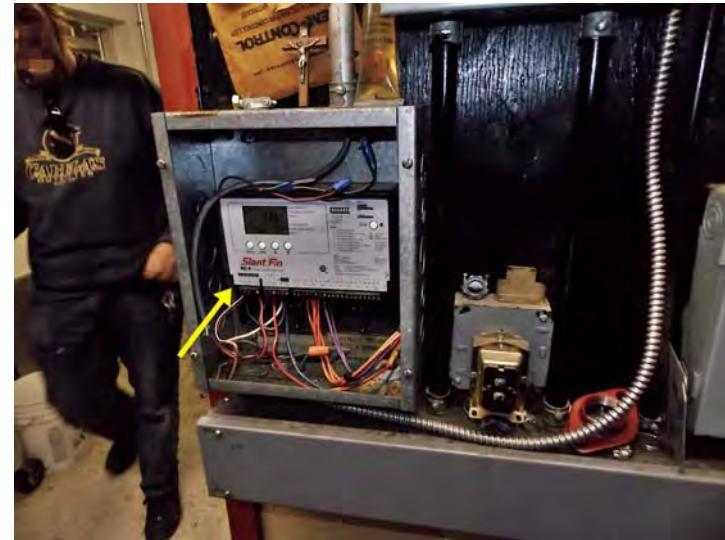
The Center's boiler plant is governed by this controller (Slant Fin).
