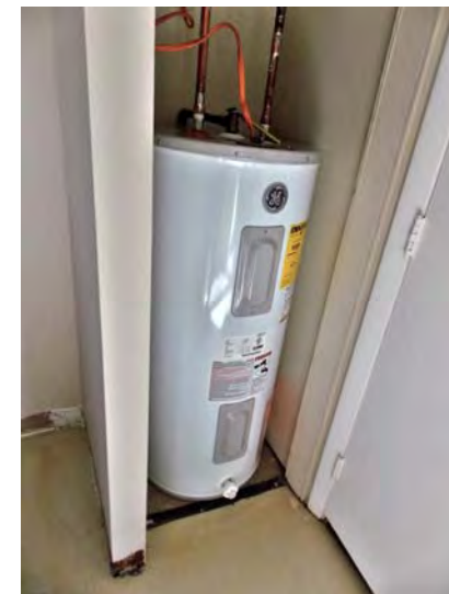
A typical electric-heated DHW tank in one of the Village's apartments.
