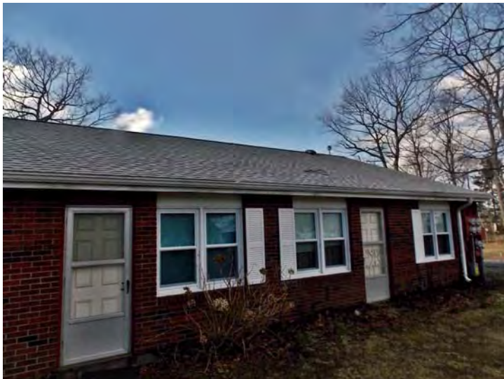
Roofs are pitched and covered with asphalt shingles.
