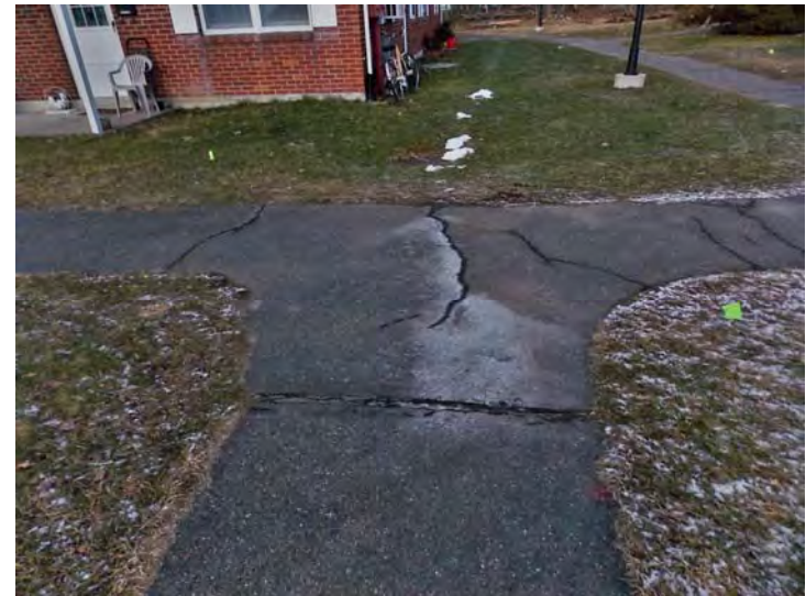
Cracks were also observed throughout the asphalt walkways.
