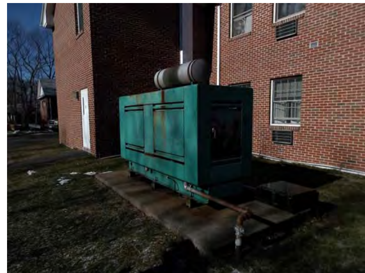
This natural gas-powered generator provides emergency power for the Center.
