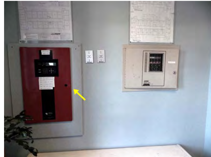
The fire alarm control system includes a newer panel (arrow). This system governs the detection devices at the Center.
