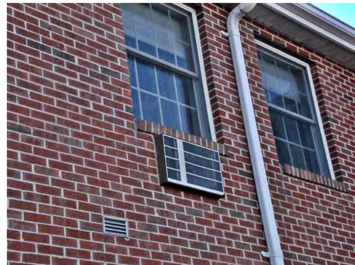
One of the air conditioner sleeves at the Center.
