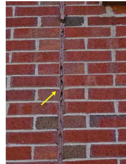
An example of dried and cracked caulking at a control joint at the Center.
