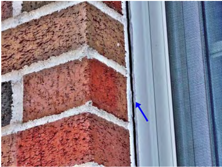
A close-up of cracked and dried caulking at a window.
