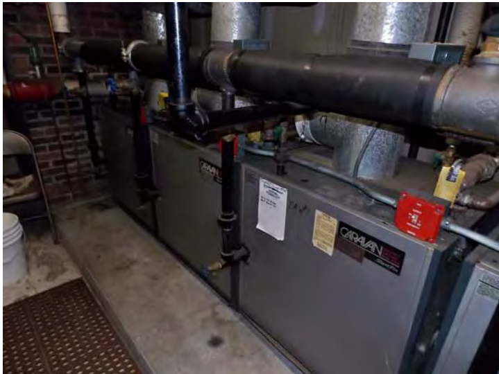
These modular boilers produce hydronic heat and DHW at the Center.
